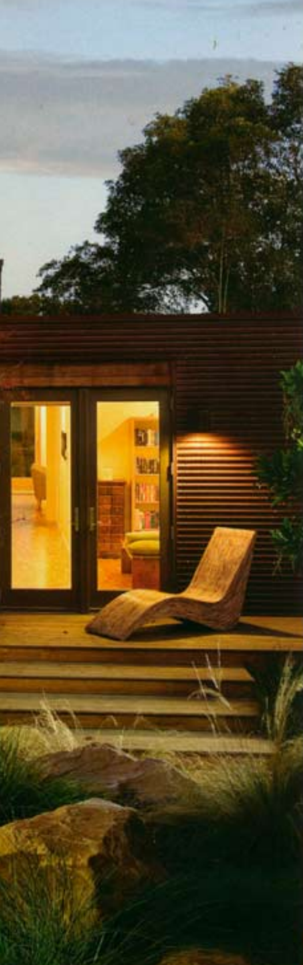
Right: The BreezeSpace opens to the front patio through large, folding glass doors. The louvered roof structure creates a changing pattern of light and shadow throughout the day.
