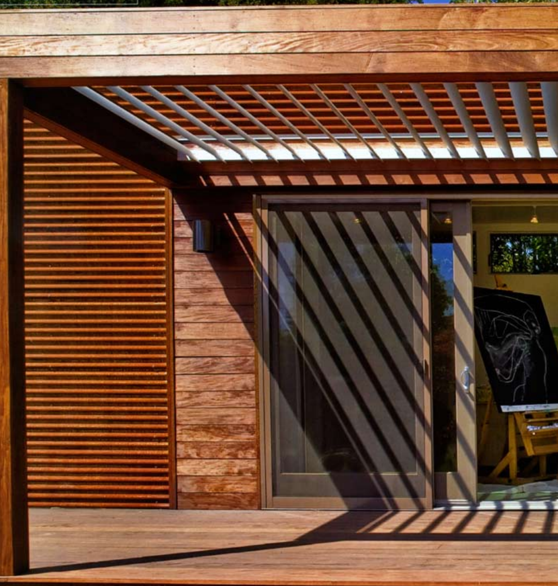
The gallery/guest house behind the main house serves as Brian Andreas' art studio. A louvered sunshade protects artwork from being damaged by direct light.
